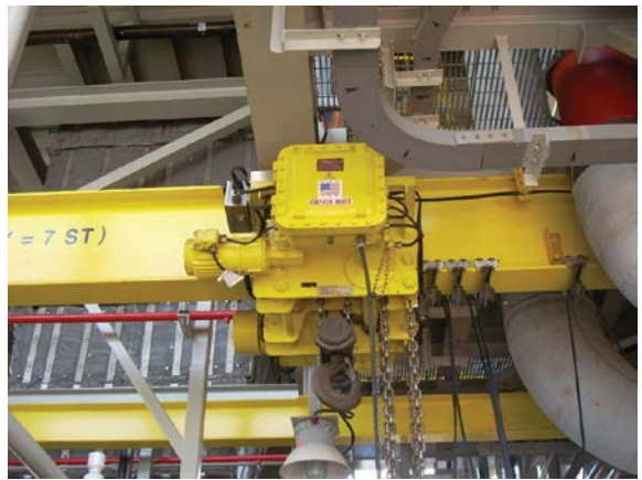
SPARK RESISTANT/EXPLOSION PROOF, 10-TON CHESTER LOW HEADROOM ELECTRIC CHAIN HOIST IN USE ON AN OFFSHORE OIL PLATFORM.
